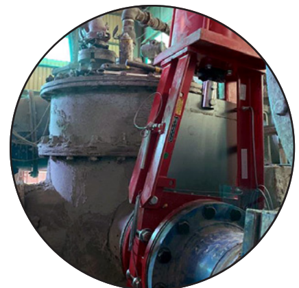
Bray Series 762 SLURRYSHIELD® knife gate valves with double-acting actuator provided 6X the service life of competitor valves.
