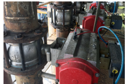
Bray's control valve packages included S19 segmented control valves with metal seats, S92 pneumatic actuators, and S6A positioners.
