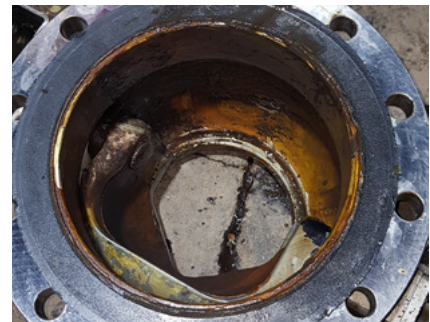
After 6 months of service, the Bray S19 valve inspection showed no signs of sugar crystal deposits, and continued trouble free service for a full 3 campaigns.
