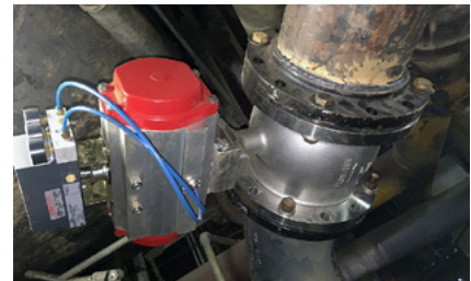
One of three automated control valve packages, consisting of an S19 segmented ball control valve, S92 double acting pneumatic actuator, and S6A positioner.
