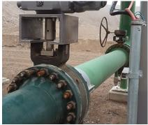
The McCannalok metal-seated double offset butterfly valve has provided more than five years of continuous service, with no failures and no maintenance required.
