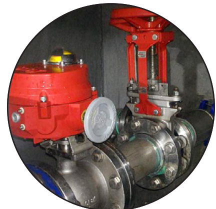
Bray knife gate valves, segmented ball control valve, and electric actuator provided absolute shutoff and precision modulation.
