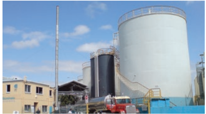
Terminals and Storage
